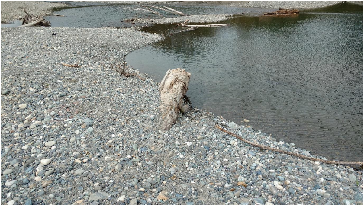
Y1(a): LWD structure (LWD# Y2016-1) placed along the bank side at downstream end of the pit in 2016 is still in place. Picture taken on August 12, 2017.
