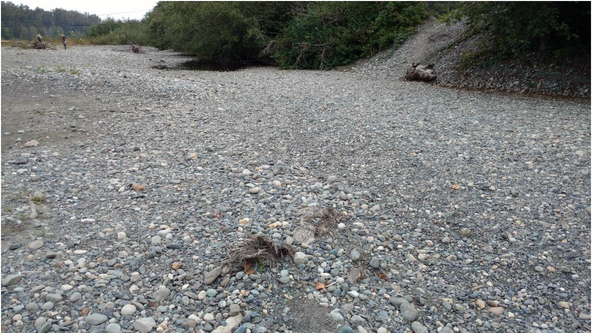
Y3(a): LWD structure (LWD# Y2016-3) placed along left-bank channel downstream of access ramp in 2016 has infilled and this part of the channel was dry at the current low flow conditions. Picture taken on August 12, 2017.
