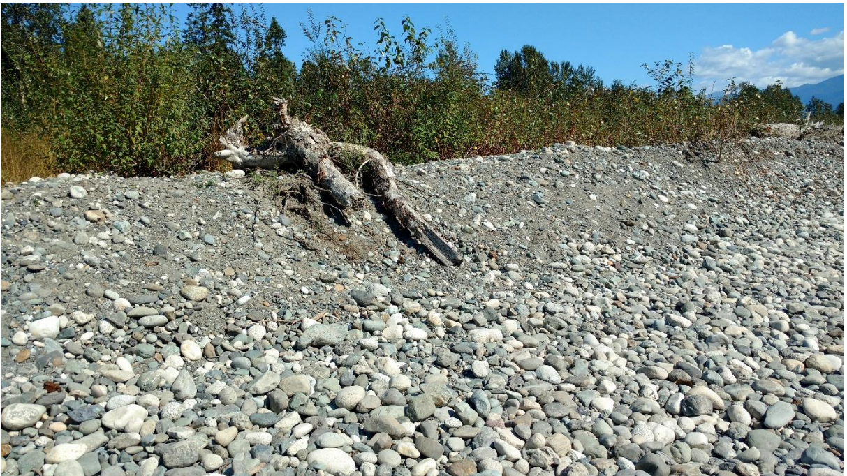
L3(a): LWD structure (LWD#L2016-3) placed along the bank-side of the pit upstream of LWD#L2016-2 in 2016 is gone. Some LWD are present on top of the bank. Picture taken on August 13, 2017.
