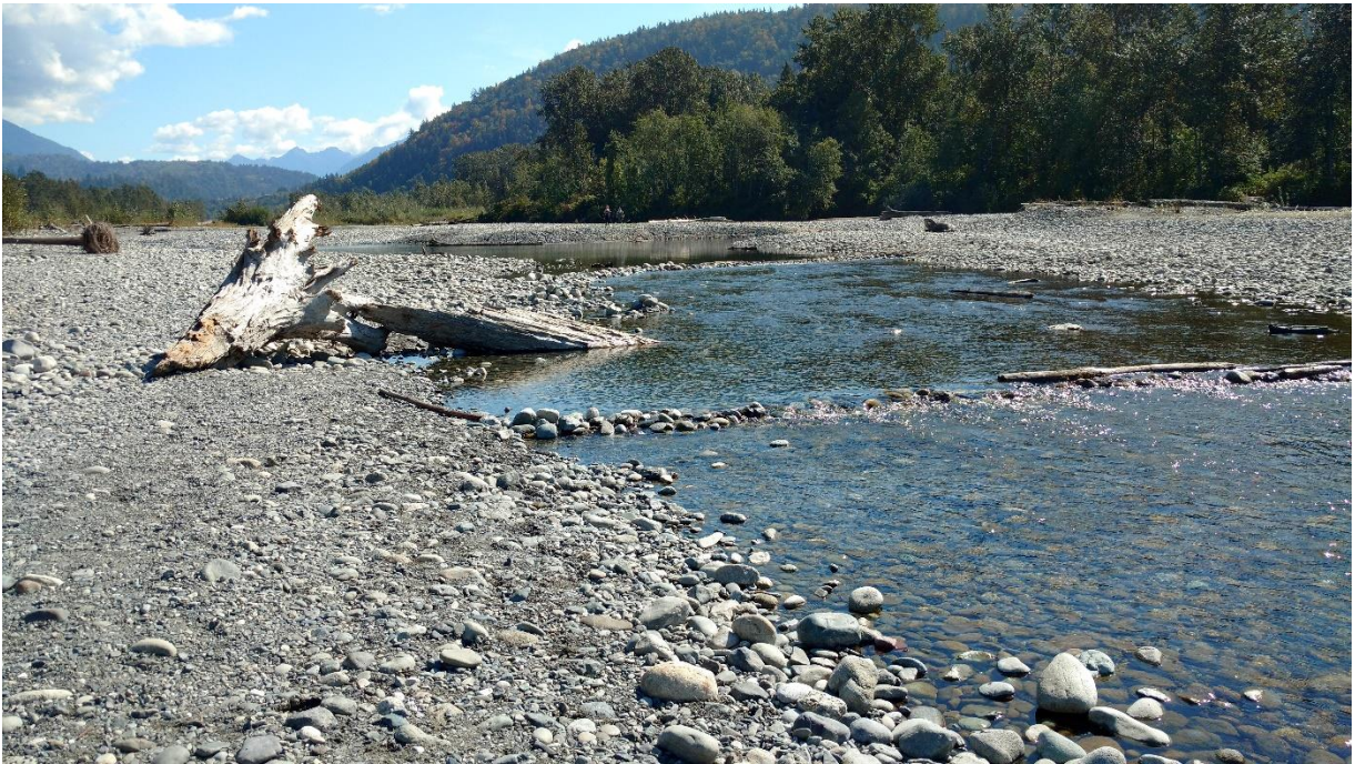
L5(a): LWD structures (LWD#L2016-5, LWD#L2016-6, and LWD#L2016-7) were placed along excavated habitat channel in 2016. Only LWD#L2016-7 is still in place. Channel attributes have improved as bed gravel has replaced previously sandy substrate. Picture taken on August 13, 2017.
