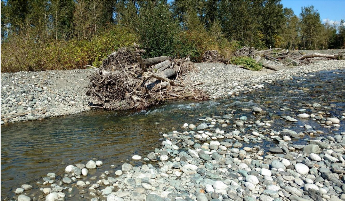
G1(a): LWD structure (LWD #G2016-1) placed in scalped pit along the channel-side in 2016 is still. The boulder platform constructed at this location may have contributed to riffle formation. Part of the river now flows through the scalped area. Picture taken on August 13, 2017.
