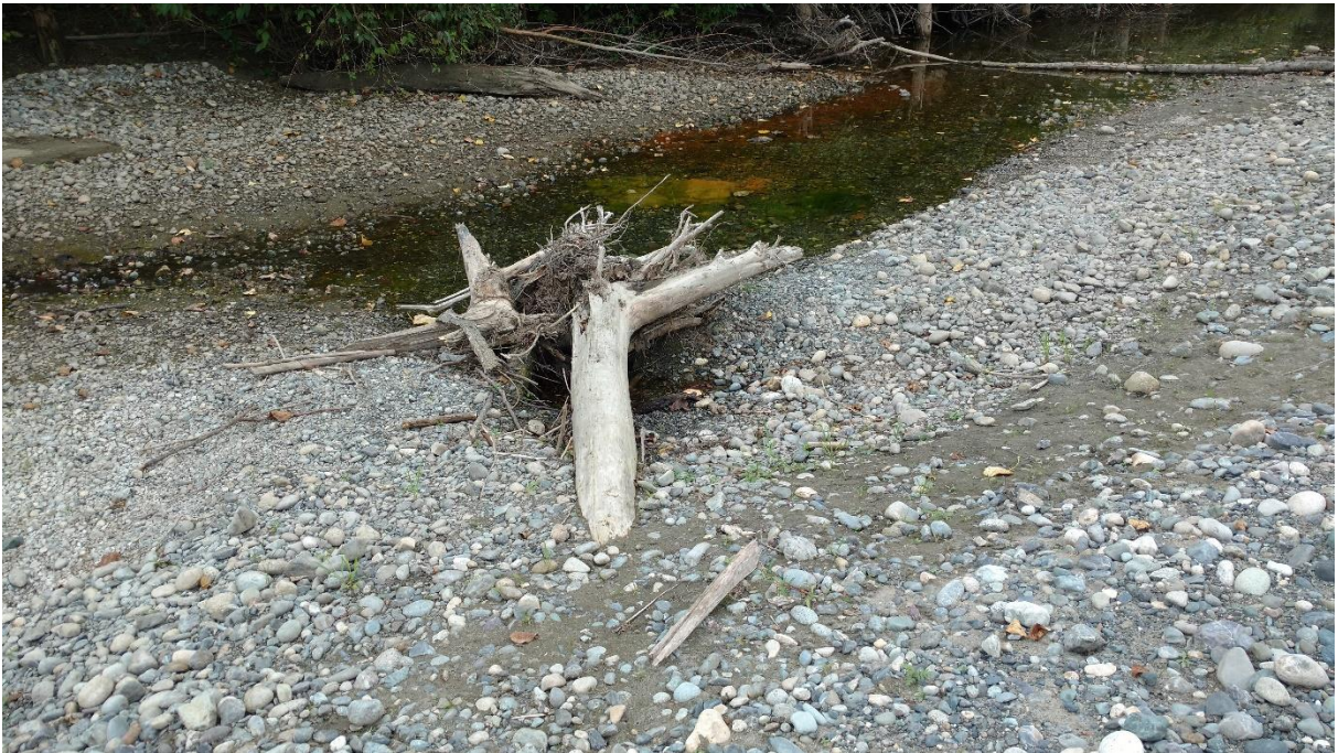
Y4(a): LWD structure (LWD# Y2016-4) placed along left-bank channel downstream of LWD# Y2016-3 in 2016 is in place. Picture taken on August 12, 2017.
