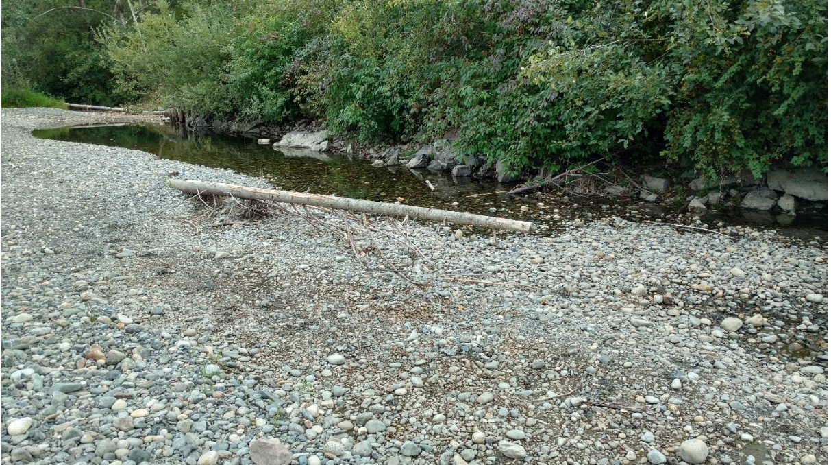
Y7(a): LWD structure (LWD# Y2016-7) placed along left-bank channel upstream of LWD# Y2016-6 in 2016 is still in place. Picture taken on August 12, 2017.
