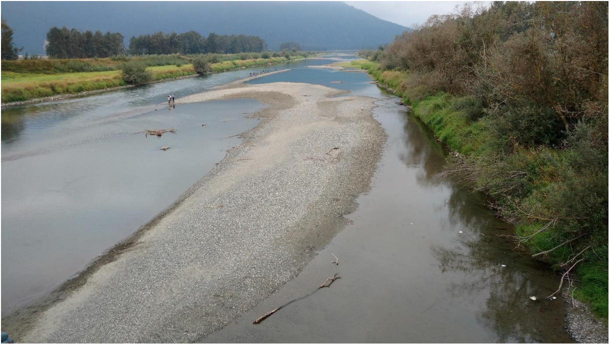
KW1(a): Excavated right-bank channel remains connected to the main flow, looking downstream from bridge. Picture taken on August 12, 2017.
