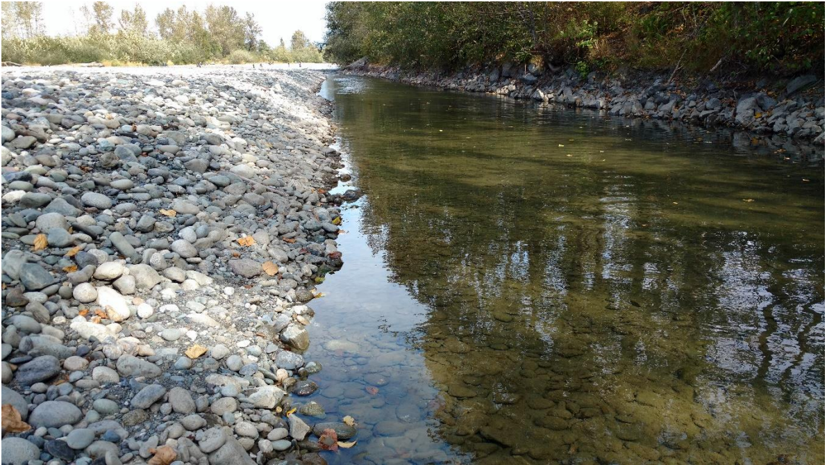
B1(a): LWD structures (LWD#B2016-1, LWD#B2016-2, and LWD#B2016-3) placed along left bank habitat channel in 2016 are gone. The habitat channel excavated along the left bank has retained both surface and groundwater flow, has supported spawning and offers a significant gain of rearing habitat. Picture taken on August 12, 2017.
