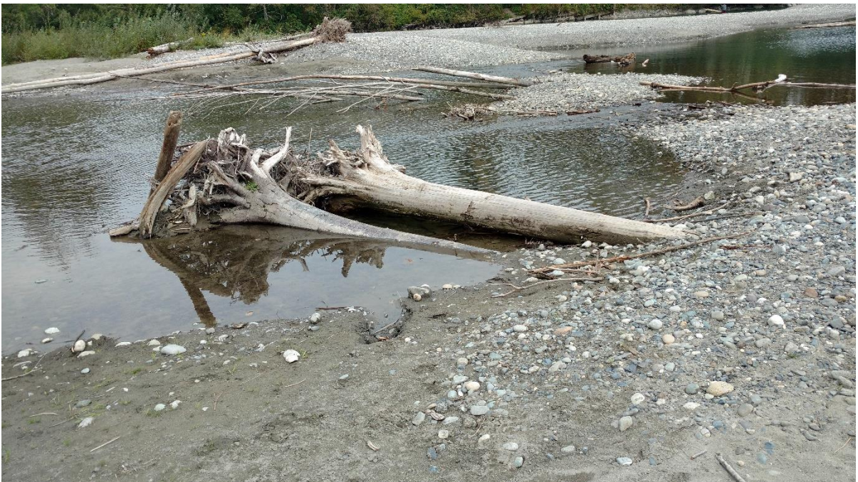
Y2(a): LWD structure (LWD# Y2016-2) placed downstream of the pit near the third opening in 2016 is still in place. Picture taken on August 12, 2017.
