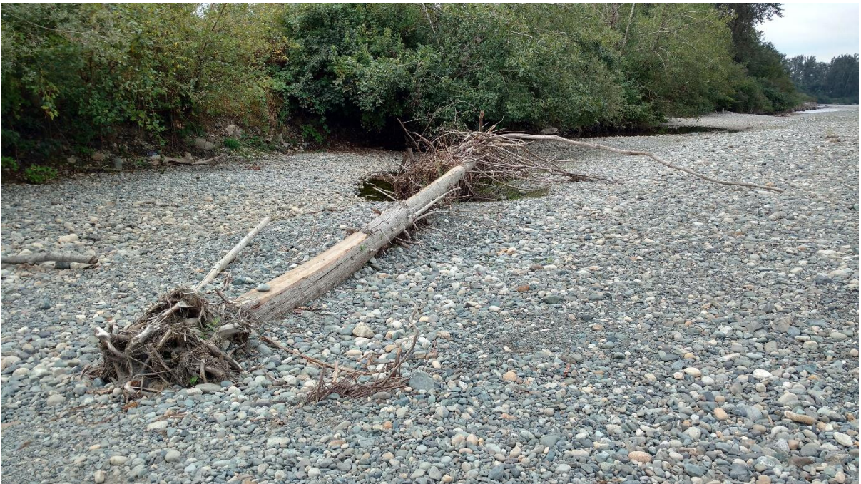
Y6(a): LWD structure (LWD# Y2016-6) placed along left-bank channel upstream of access ramp in 2016 is still in place. Picture taken on August 12, 2017.
