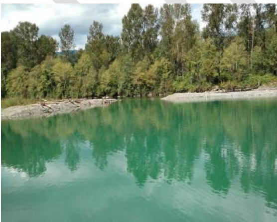
Y11: View of the completed excavation, looking towards outflow opening. September 10, 2016.
