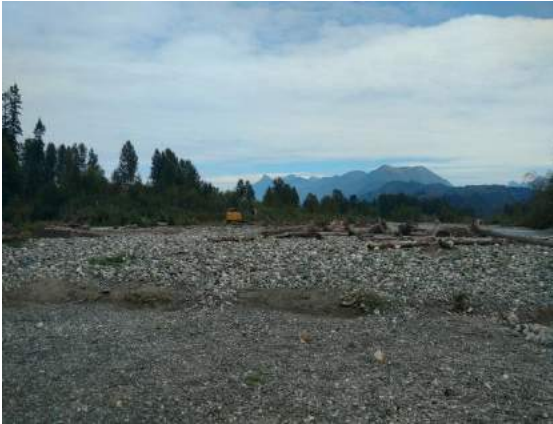
L1: Lickman sediment removal site prior to work facing upstream. September 9, 2016.
