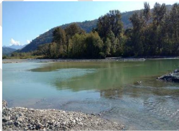
L10: View of the completed excavation from downstream of the work, near second outflow to the constructed channel. September 27, 2016.
