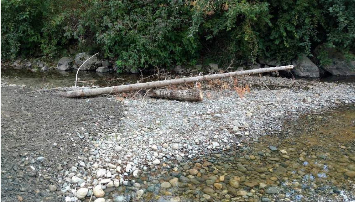
Y7: LWD #Y2016-7 –LWD structure placed along left bank side channel upstream of LWD #Y2016-6.
