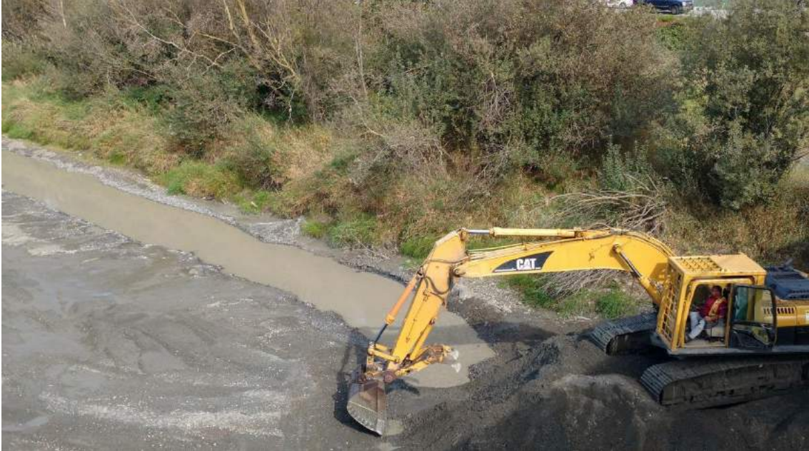
Construction of a habitat channel along the right bank. September 29, 2016.
