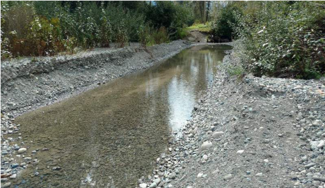
Completed upstream habitat excavation. View towards left bank side channel. September 10, 2016.
