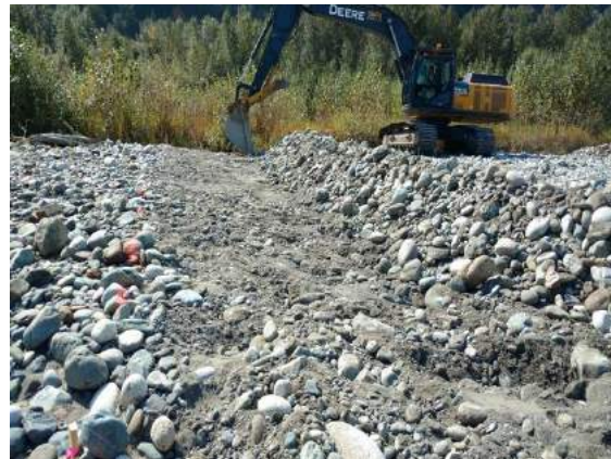
G6: Beginning of excavation at upstream end with 10:1 slope. August 10, 2016.
