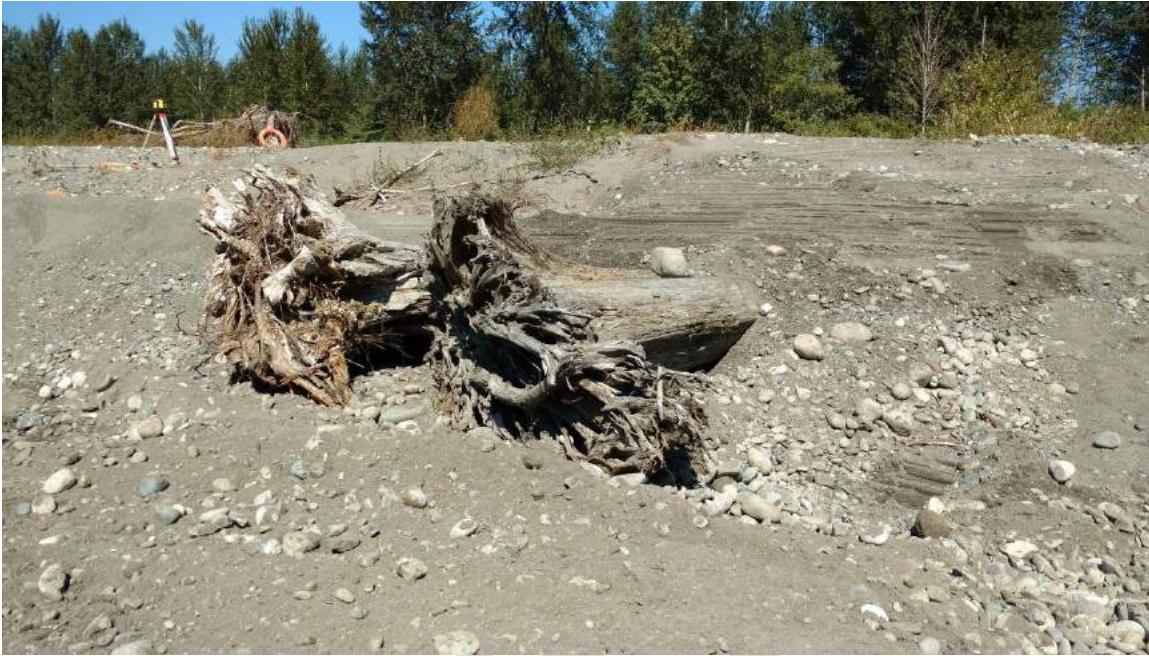
G1: LWD #G2016-1 – two pieces of LWD placed in scalped pit along the river side.
