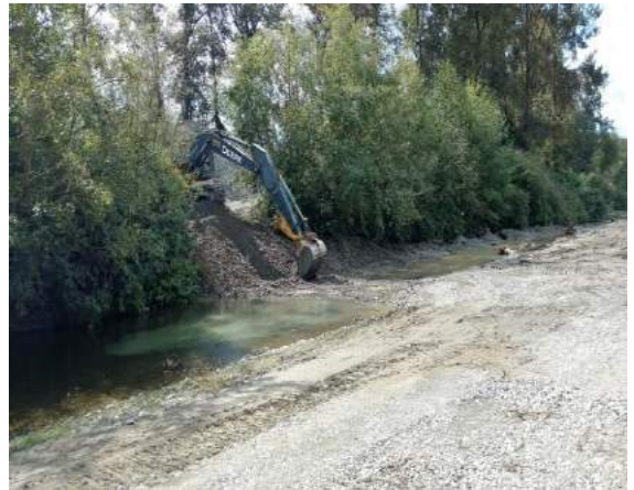
Y12: Restored channel after access road decommission. September 8, 2016.
