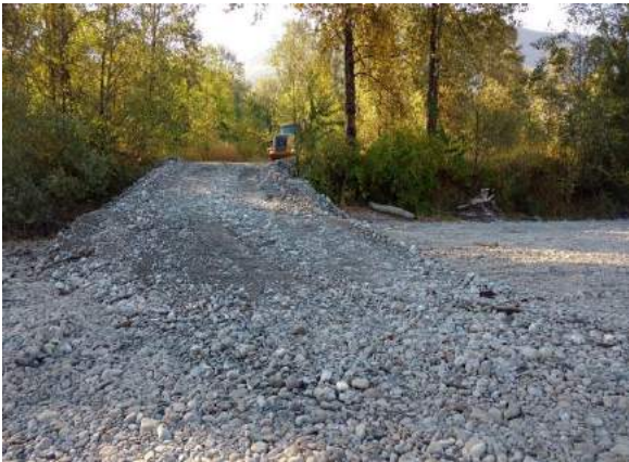
B3: Access road constructed. August 18, 2016.
