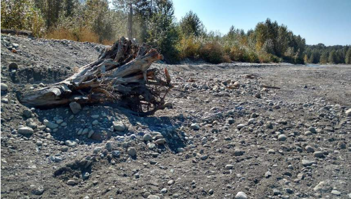
G3: LWD #G2016-3 – two pieces of LWD placed in scalped pit along the bank side. Note a platform of boulders created downstream of LWD complex to enhance fish habitat.
