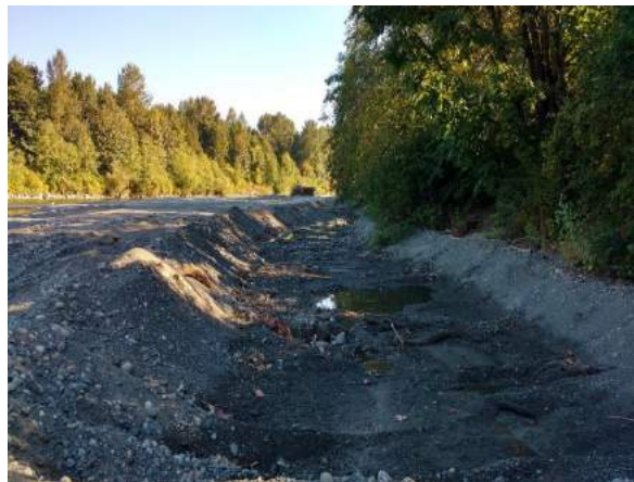
B6: Habitat channel construction. August 23, 2016.
