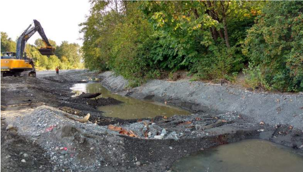
Habitat channel construction work in progress looking upstream. August 26, 2016.
