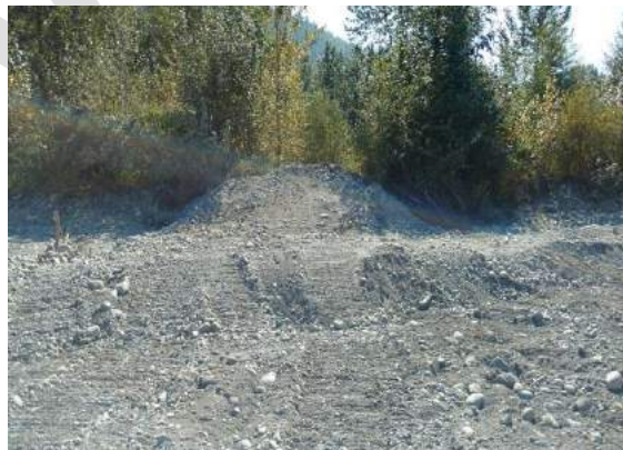
G12: Restored access to the bar after access ramp decommission. August 17, 2016.
