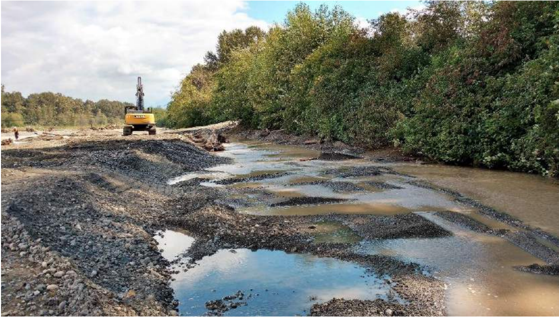
Left bank side channel widening. View upstream. September 8, 2016.
