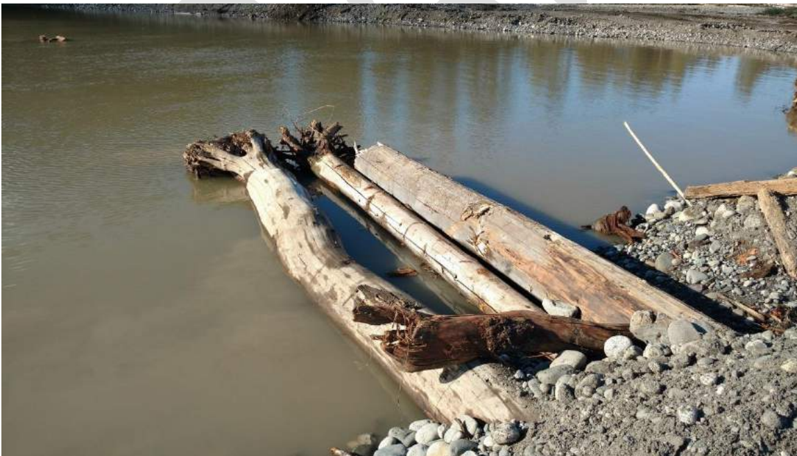
L2: LWD #L2016-2 –LWD structure placed along the bank side of the pit upstream of LWD #L2016-1.
