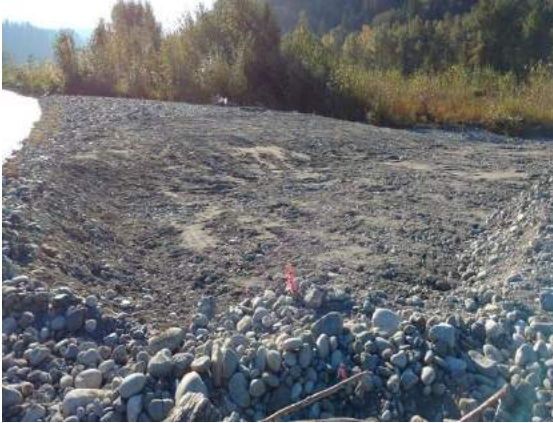
G7: Gradual slope transition at upstream end of excavation. August 11, 2016.
