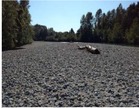
B2: Bergman sediment removal site prior to work facing downstream. August 17, 2016.
