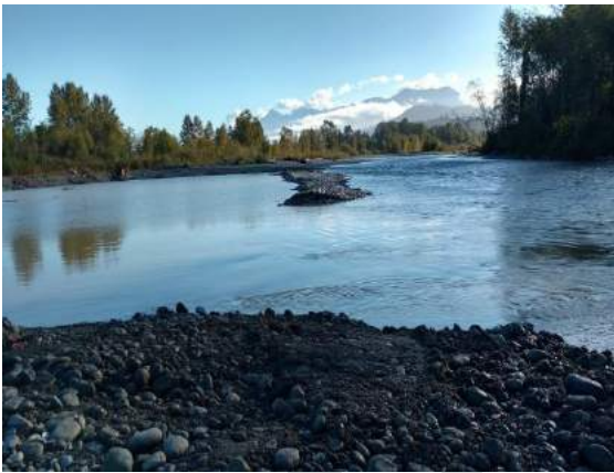
L9: Outflow of completed site. September 27, 2016.
