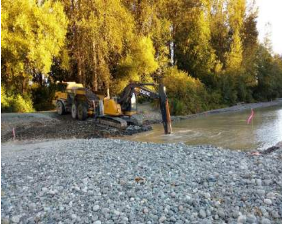
R7: Downstream end completion with 1.5:1 slope. September 13, 2016.
