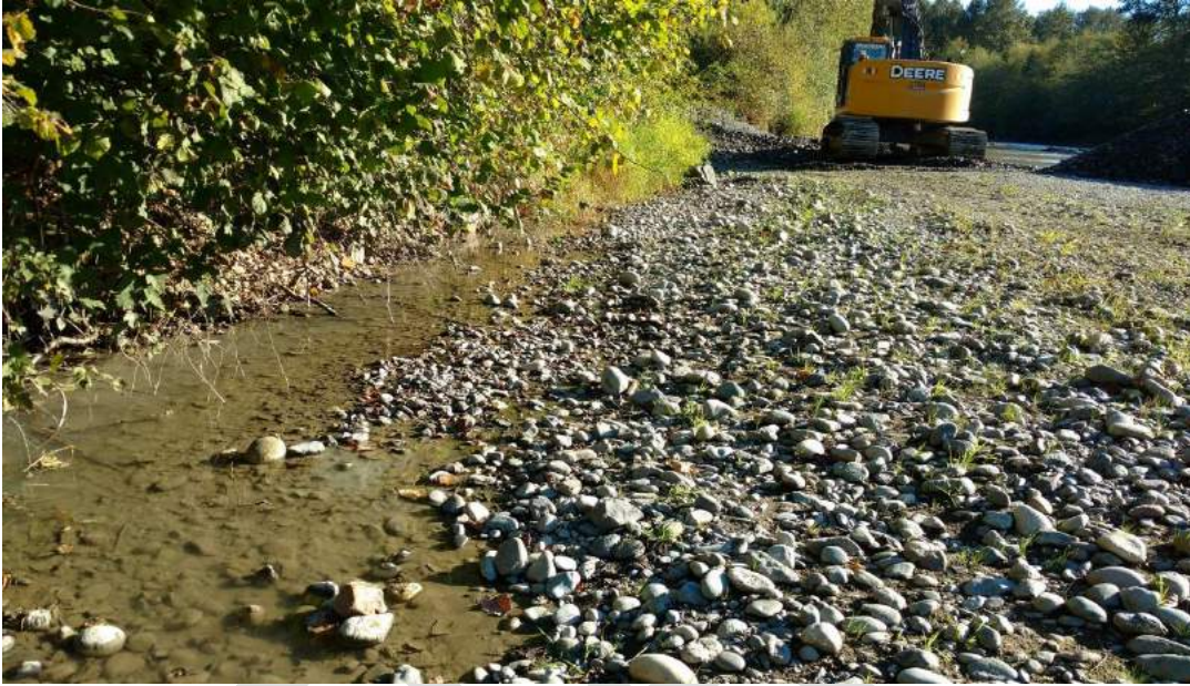
Right bank side channel before enhancement, looking upstream. August 13, 2016.
