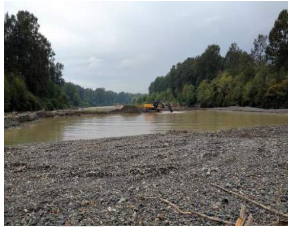
Y8: Work in progress. View from upstream end of site. September 7, 2016.
