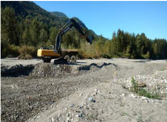
G9: Work near completion at downstream end of excavation. August 16, 2016.
