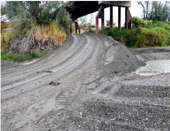
KW3: Bar access ramp constructed. September 6, 2016.
