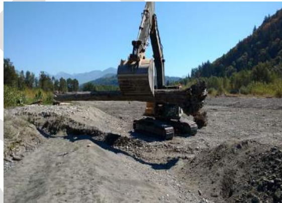
G10: LWD placing along the river side of the pit. August 17, 2016.
