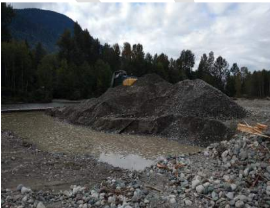
L5: Beginning of excavation at upstream end with 5:1 slope. September 10, 2016.
