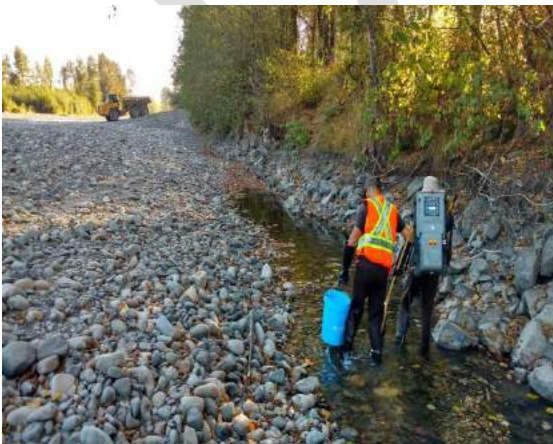
B5: E-fishing prior to channel construction. August 19, 2016.
