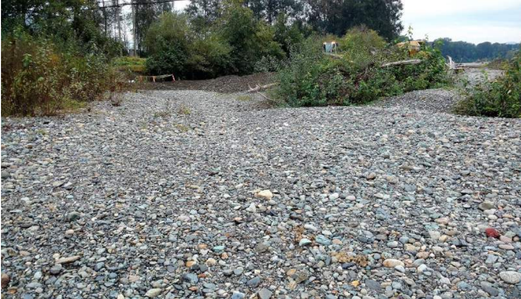
Upstream excavation site prior to work. September 7, 2016.
