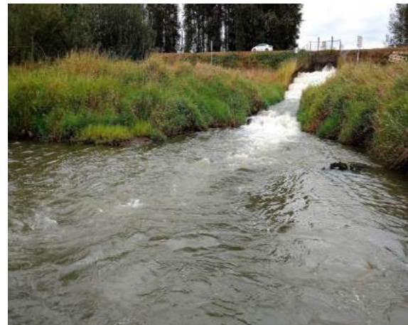
KW6: Pump station water release. September 7, 2016.
