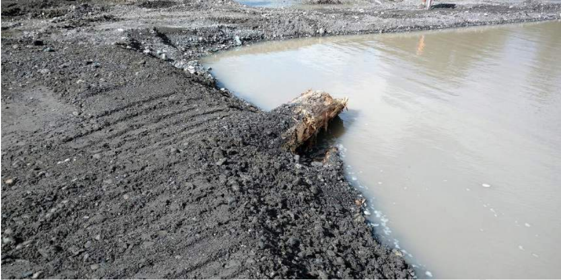
Y1: LWD #Y2016-1 – one piece of LWD placed along the bank side at downstream end of the pit.
