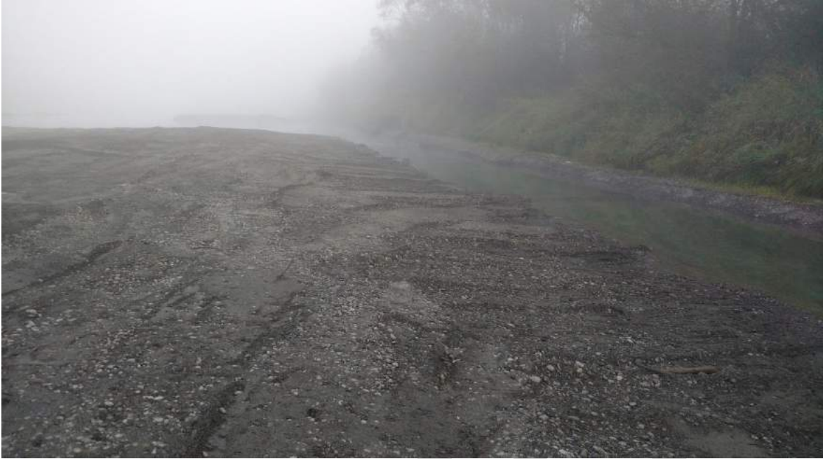
Habitat channel completed, looking downstream. September 30, 2016.
