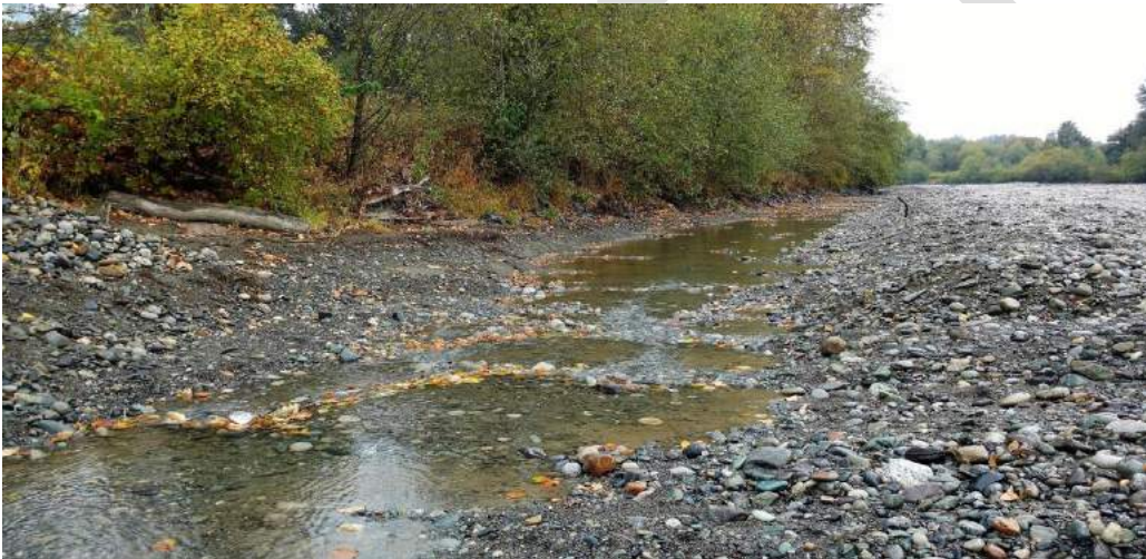
Completed habitat channel looking downstream. August 31, 2016.
