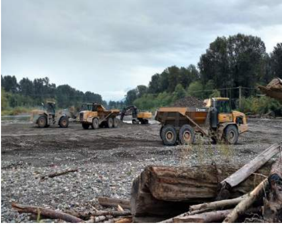
Y7: View of machinery and work activities on site. August 31, 2016.
