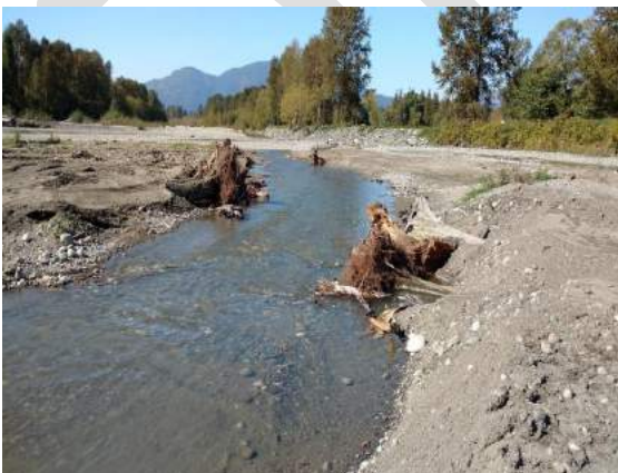
L11: Constructed channel, view downstream. September 27, 2016.
