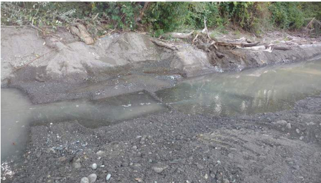
Habitat channel construction. Pools and riffles structures applied. August 26, 2016.
