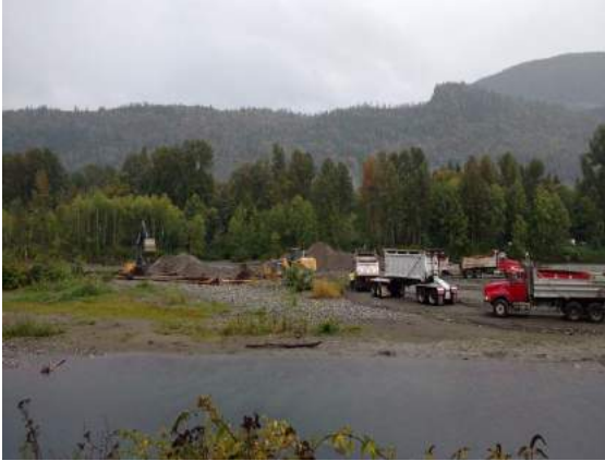
L7: Machinery on site. September 19, 2016.
