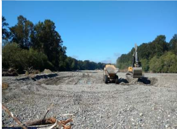
Y4: Scalping of deep pit area. August 29, 2016.
