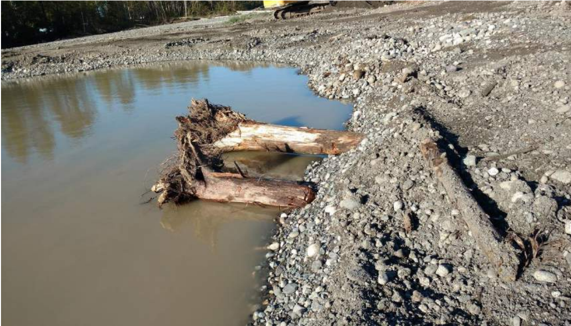
L1: LWD #L2016-1 –LWD structure placed along the bank side of the pit.
