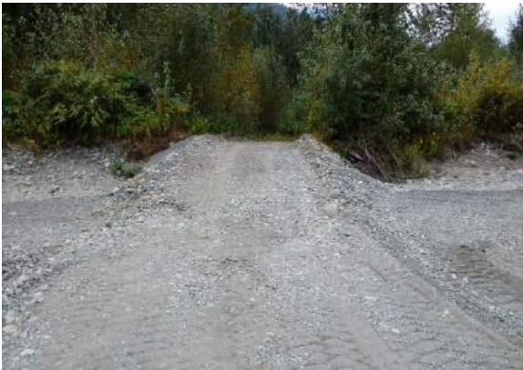
G3: Access ramp constructed. August 9, 2016.
