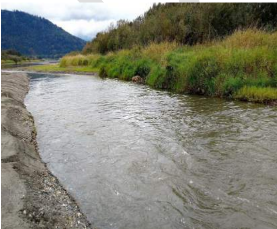
KW5: Pump station outflow channel constructed. September 7, 2016.
