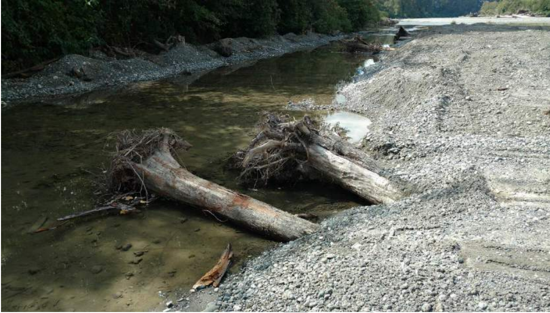
Y3: LWD #Y2016-3 –LWD structure placed along left bank side channel downstream of access ramp.
