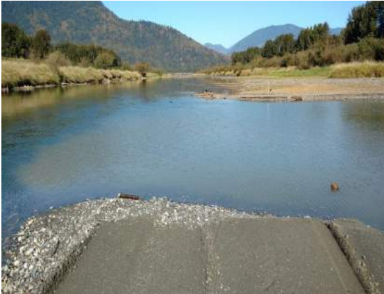
KW9: Constructed outflow opening to the main river. September 28, 2016.
