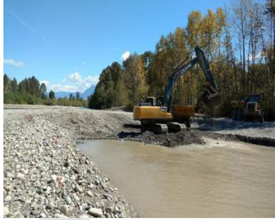
B8: Upstream end completion with 5:1 slope. August 25, 2016.
