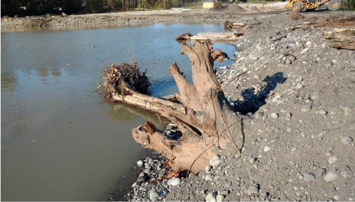
L3: LWD #L2016-3 –LWD structure placed along the bank side of the pit upstream of LWD #L2016-2.
