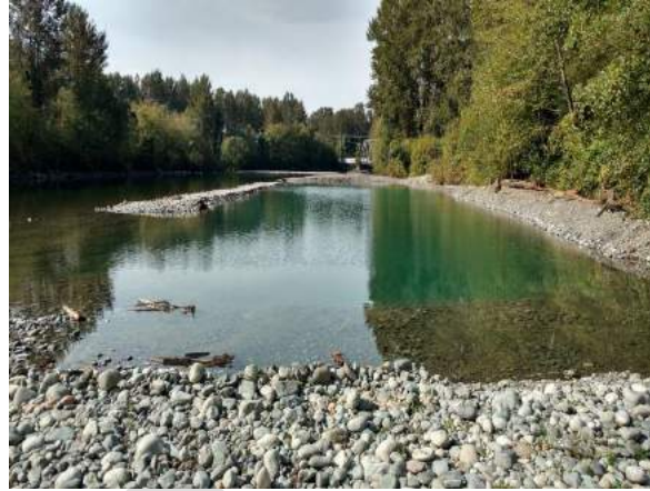
R8: Inflow of the completed site. September 16, 2016.
