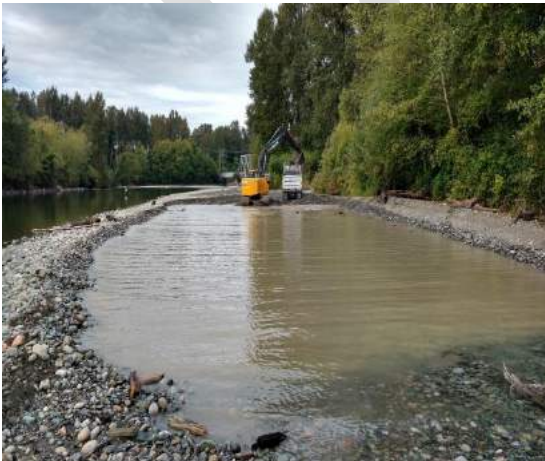
R5: View of work activities from upstream end of site. September 10, 2016.
