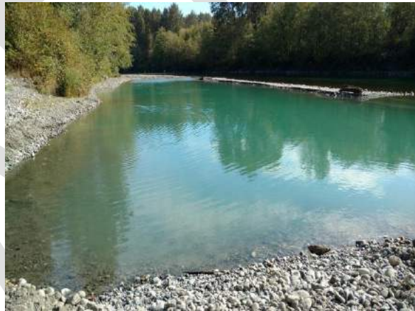
R10: View of the completed excavation from the downstream end. September 16, 2016.
