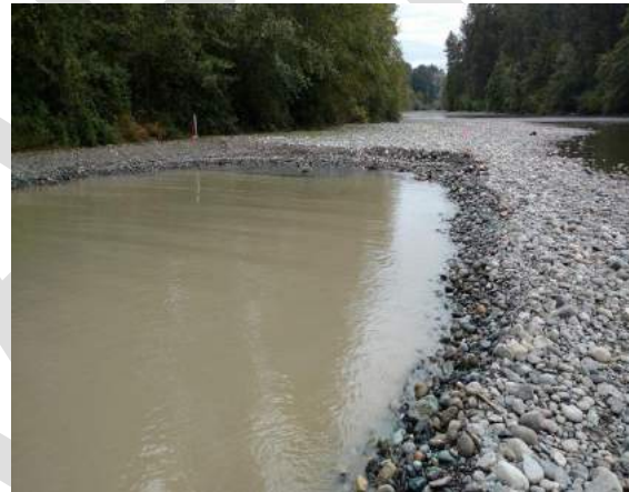
R4: Beginning of excavation at upstream end with 5:1 slope. September 10, 2016.
