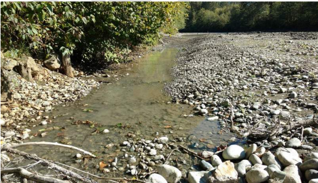
Right bank side channel after enhancement, looking upstream. August 13, 2016.
