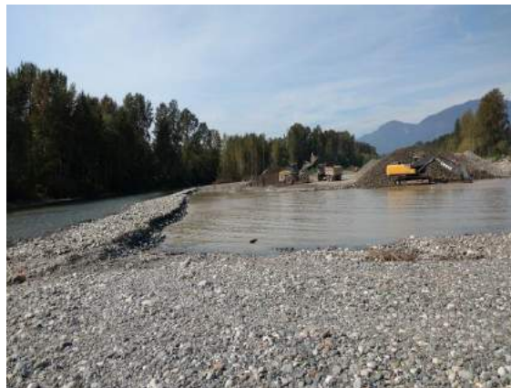
L6: Ongoing work activities: view from upstream part of excavation. September 13, 2016.
