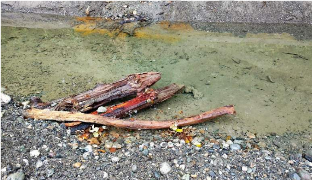
B2: LWD #B2016-2 –LWD structure placed along left bank habitat channel upstream of LWD #B2016-1.
