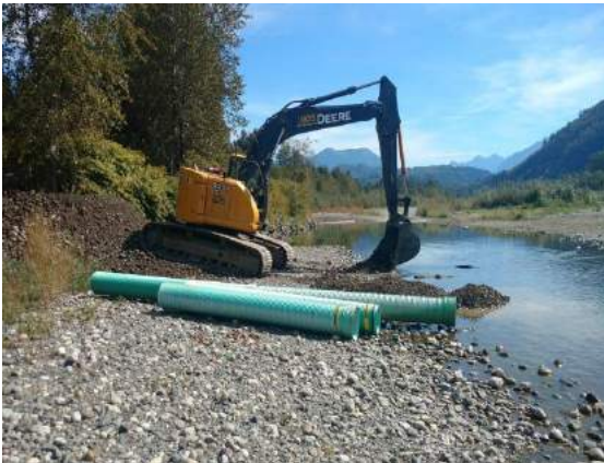
L3: Installation of site access ramp. September 9, 2016.
