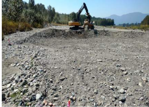
G8: View of work activities from upstream end of site. August 11, 2016.
