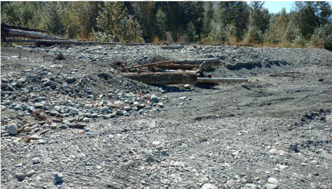
G2: LWD #G2016-2 – several pieces of LWD placed in scalped pit along the bank side. Note a platform of boulders created upstream of LWD complex to enhance fish habitat.
