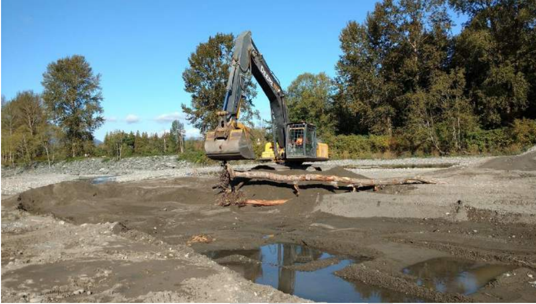
Habitat channel construction and placement of LWD. September 27, 2016.
