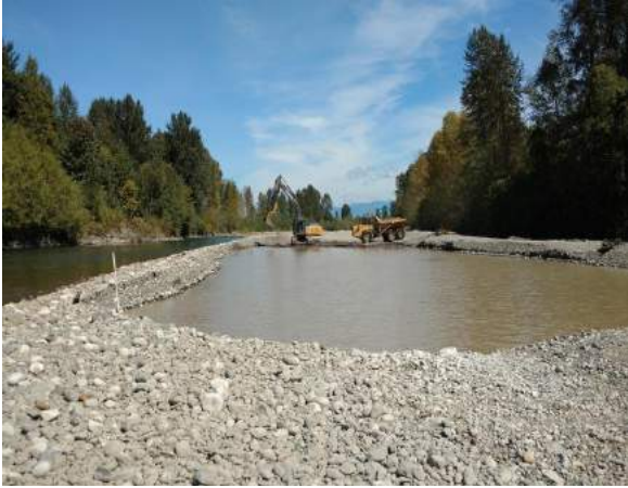
B7: View of work activities from downstream end of site. August 24, 2016.
