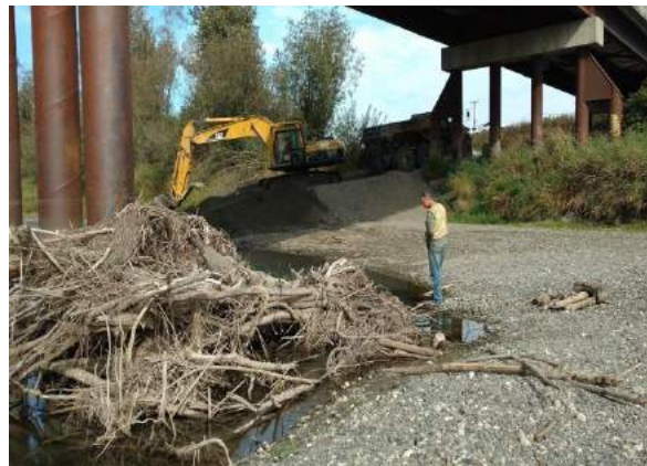
KW12: Access road decommissioning. September 29, 2016.
