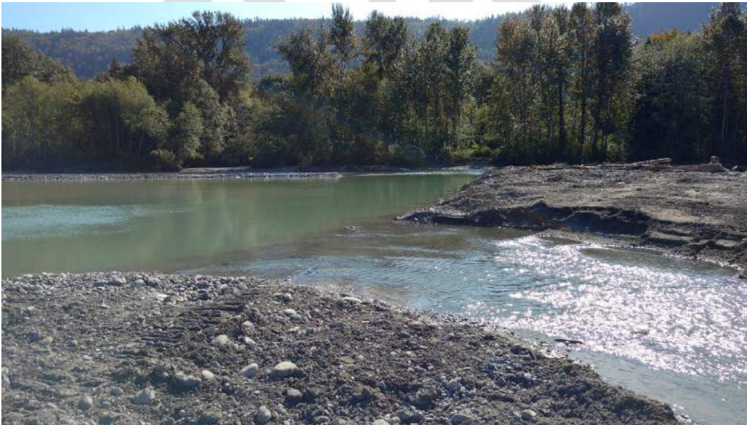
Deep pit outflowing into newly constructed habitat channel. September 27, 2016.
