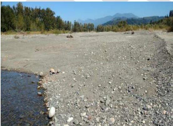
G11: View of the completed excavation from downstream of the work. August 17, 2016.
