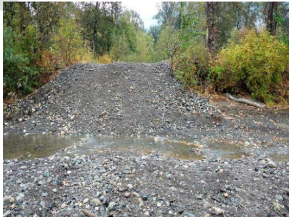
B12: Restored channel after access road decommission. August 31, 2016.
