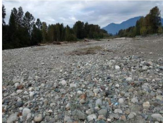
L2: Lickman sediment removal site prior to work facing downstream. September 9, 2016.
