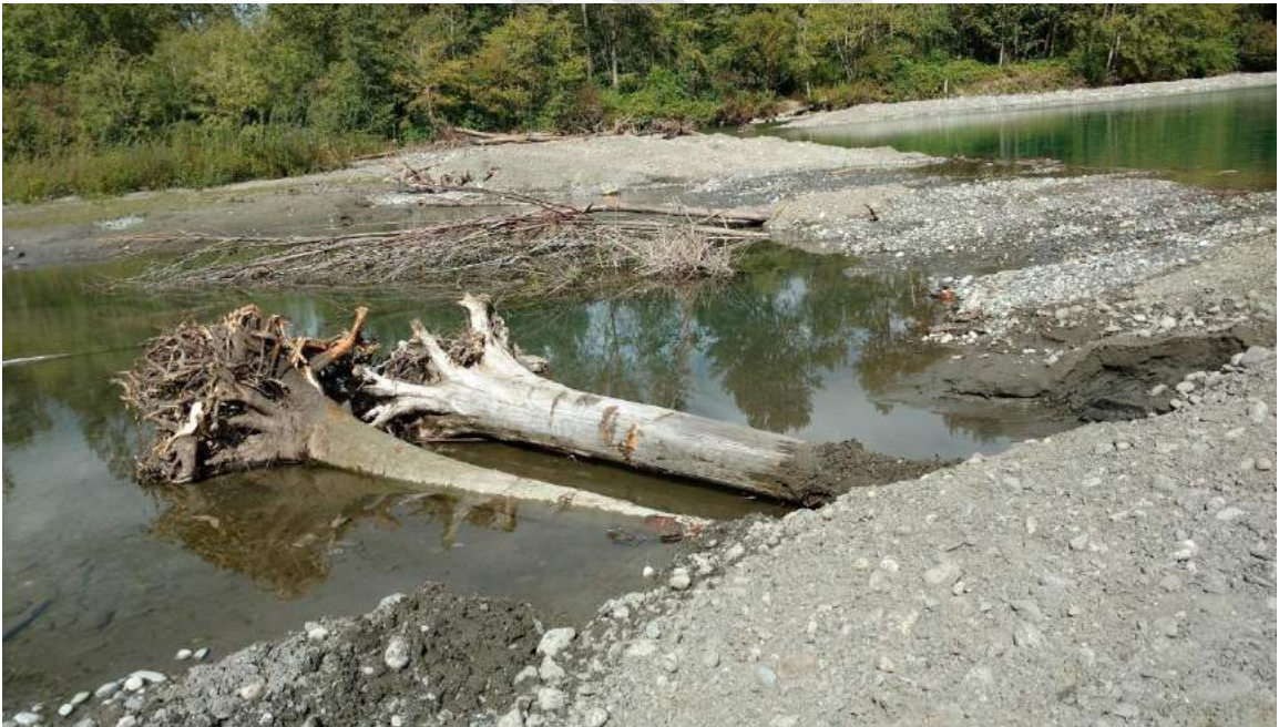
Y2: LWD #Y2016-2 – two pieces of LWD placed downstream of the pit near the third opening.
