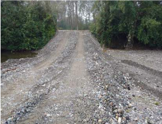
Y3: Bar access ramp constructed. August 29, 2016.
