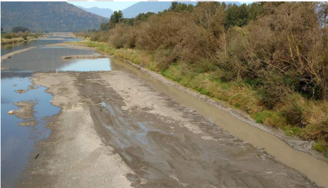
Habitat channel connected to the pit, looking from upstream of work. September 29, 2016.
