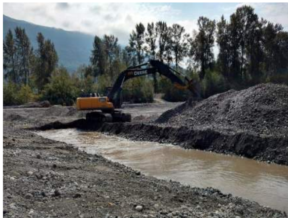
Y6: Start of excavation at upstream end with 5:1 slope. August 30, 2016.
