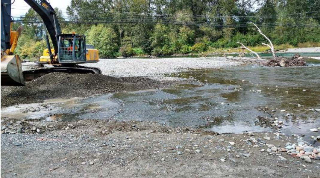
'Riffle structure' connection to the river at the upstream end of habitat excavation. September 8, 2016.
