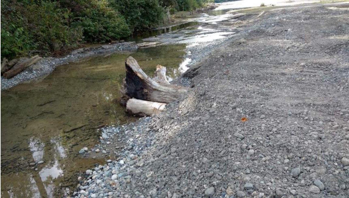
Y5: LWD #Y2016-5 –LWD structure placed along left bank side channel downstream of LWD #Y2016-4.
