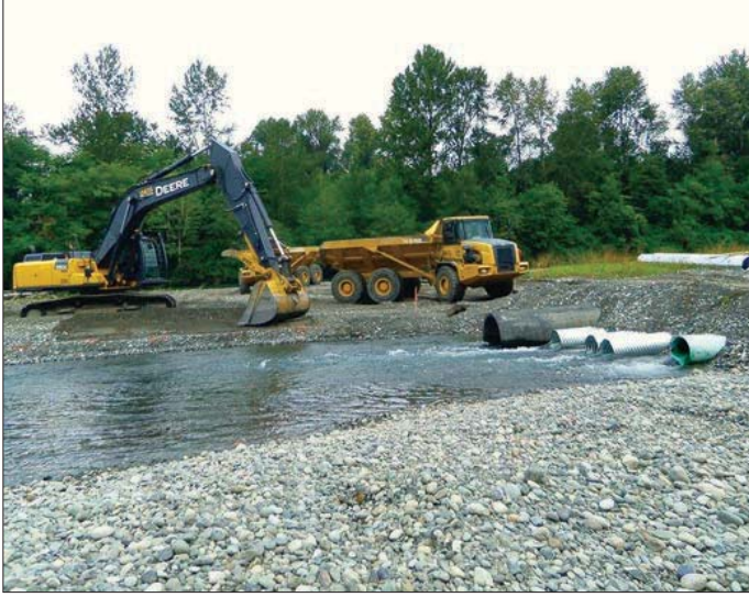
Sediment is removed, 2014.
