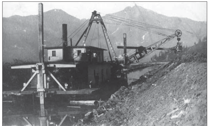
TOP: Vedder River, early 1900s; BOTTOM: The canal is dredged to divert Vedder River into the Sumas River.
